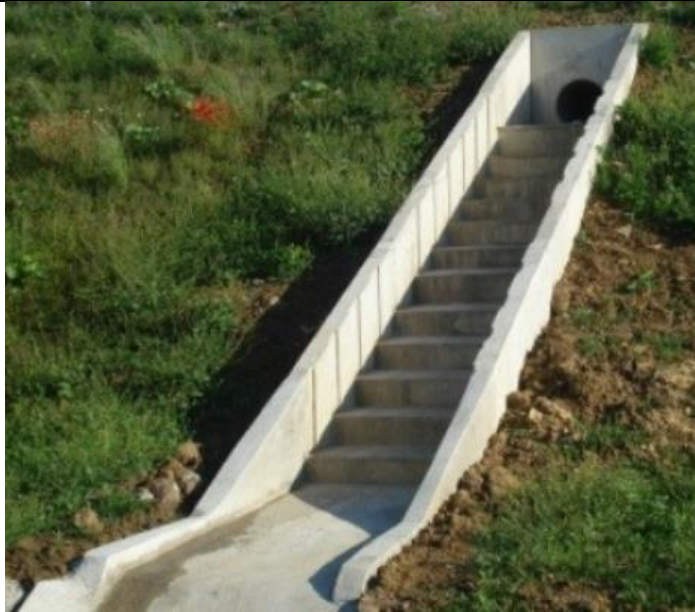
Staircase energy breaker on road embankment
