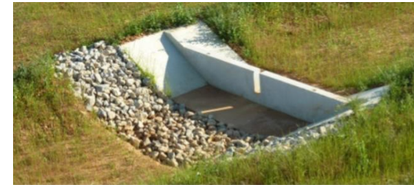
Cascading overflow structures on a ditch( view from downstream)
