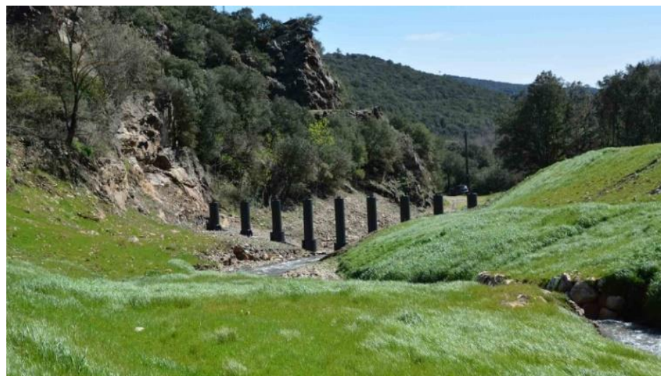
Trash Combs upstream of Bridges and Culverts
