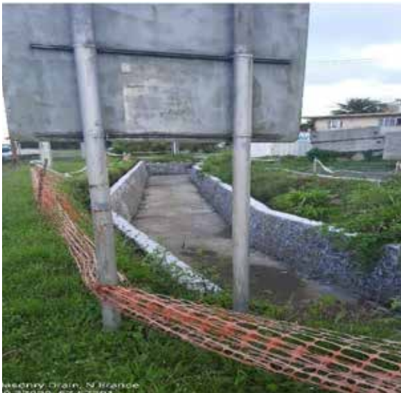
1.Construction of trapezoidal masonry drain (Alignment 3)
