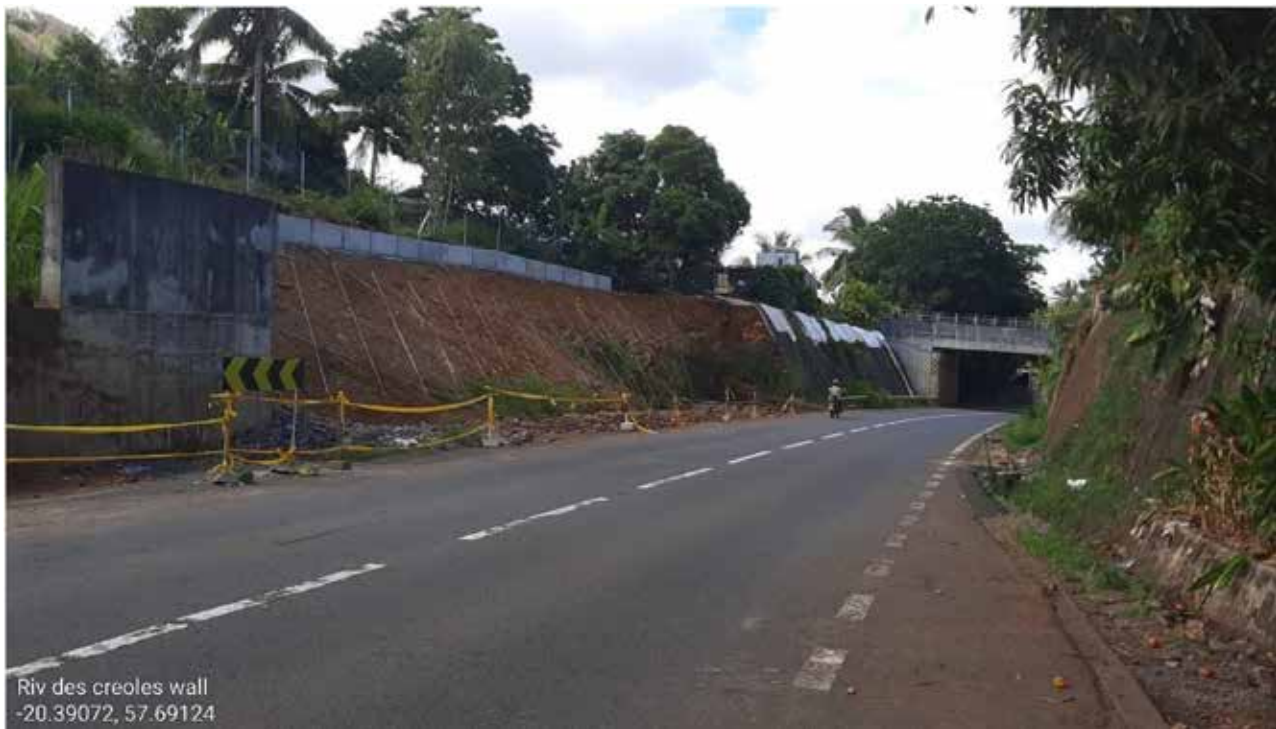
Construction of RC parapet wall along diverted drainage path at Riv des creoles
