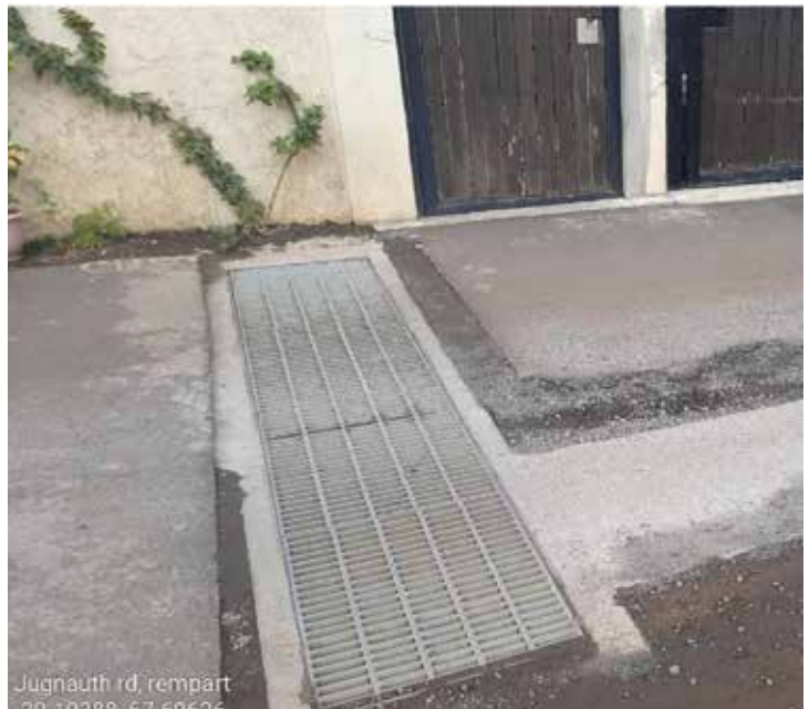
9. Rivière du Rempart-Construction of absorption drain nr Musligadoo at bend in first Lateral, Ext Jugnauth Road
