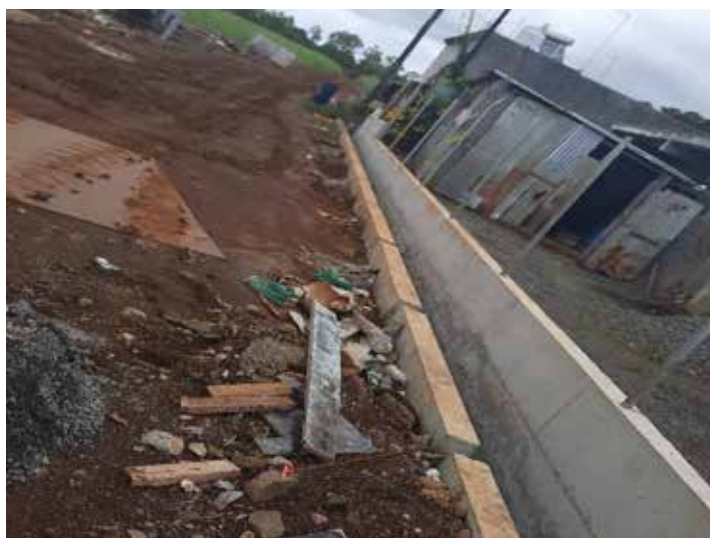
Amaury- Cut off drain in the region of Cemetery & Cite EDC Amaury
