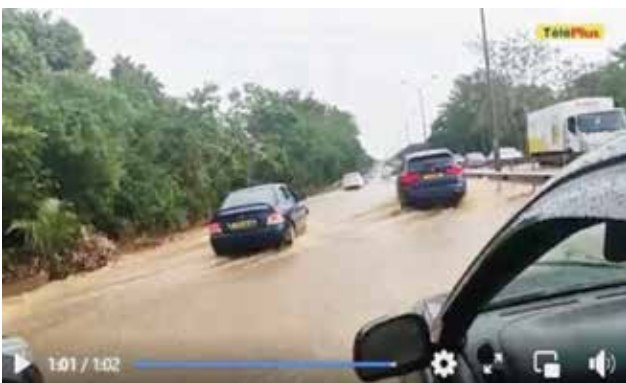
Water accumulation on RDA Motorway Near Pamplemousses Provision of roadside drains and reprofiling of road towards the roadside drain.
